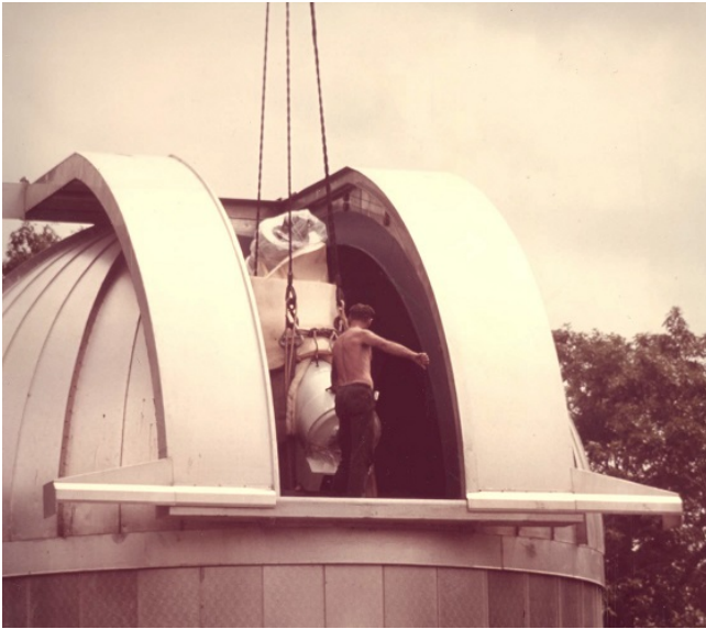
Figure 2. 16-inch telescope installation. Here we see, during installation in 1971, a crane guiding the Ealing 16-inch mount into place where it would live for 46 years.
